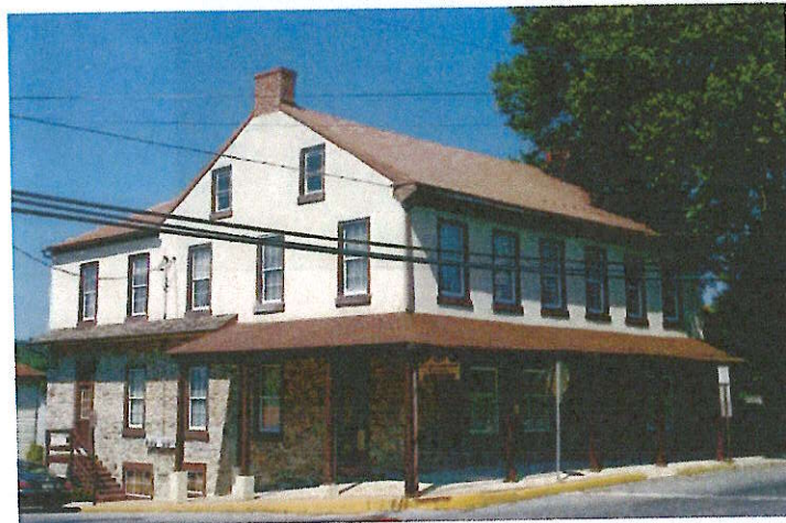
Architectural details include front porch and dual brick chimneys.
