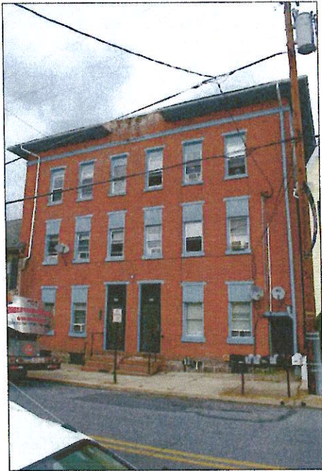
Various utilities are in public view that could be relocated to be less visible.
