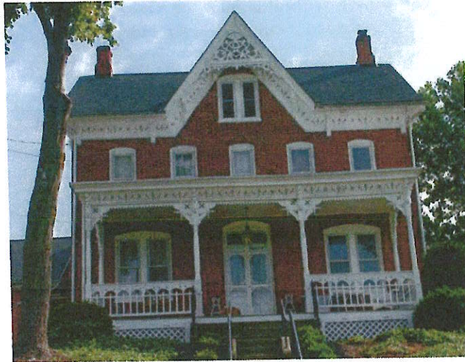
Victorian structure exhibits character-defining architectural details such as cornices, lintels, balustrades and dual brick chimneys.
