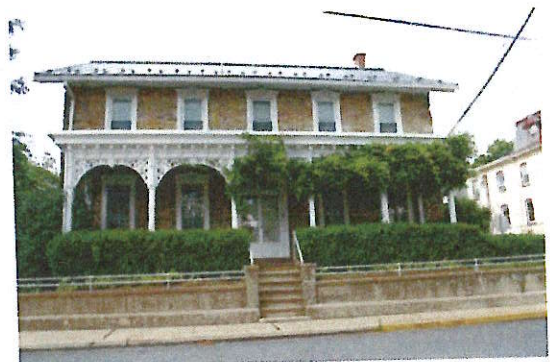
Retaining wall and fence define a wall of continuity
