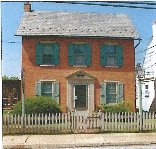
Wooden picket fence with gate used to delineate a front yard, painted to match trim on building
