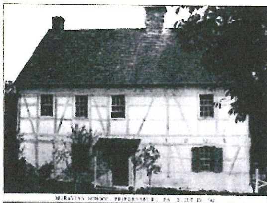
An early photo of the Moravian boarding school, built in 1742, and now the victim of deterioration and demolition. The half-timber construction was unique and there are no other remaining examples known in the township or in Berks County.
